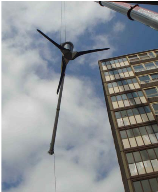
Lifting the wind turbine onto the roof © Photon Energy
