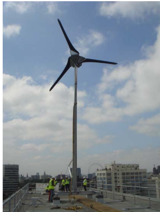
Wind turbine installation nearing completion © Photon Energy
