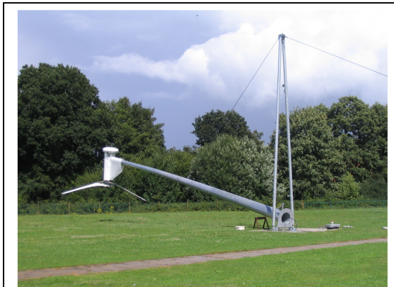
Installation of the 6 kW wind turbine at Maidenbower Junior School
