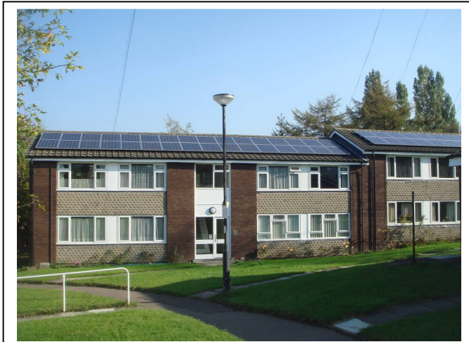
Blocks of flats with PV
