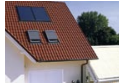
Family house with solar thermal system for hot water supply
