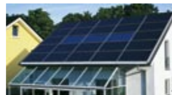
complete roof installation
