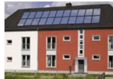
Apartment building with solar thermal system for auxiliary heating
