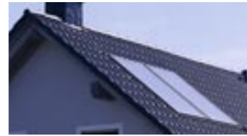
In-roof and complete roof installation
